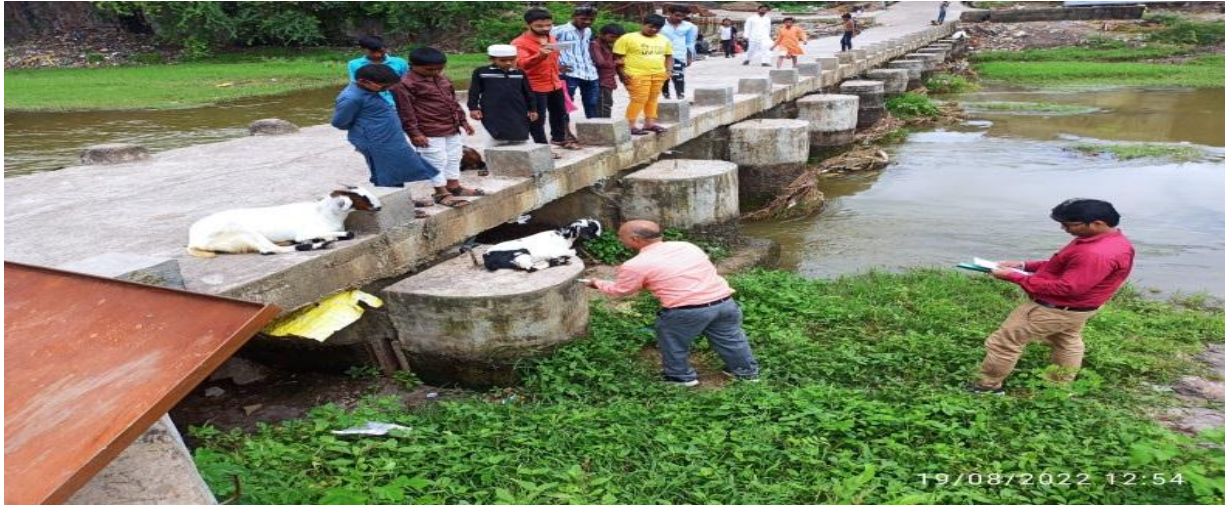
Bridge Site at M.C. Balapur
